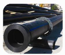
(4) **Flanges** are placed at the ends of the 65 m sections.
