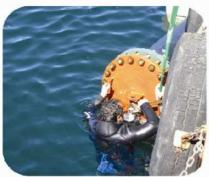
(10) With the help of a scuba diver, a pressure gauge and a valve are placed on the pipe end which has not been joined. First of all, pressurised air is introduced until it is balanced with the water pressure.
