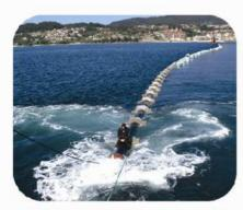
(12) The pipe is filled with potable water, which begins the sinking process up to the end with the flange, through which air from inside the pipe is pushed out. The aim is that sinking takes place with a radius of curvature as broad as possible, in order to prevent the joined parts from suffering during the process.
