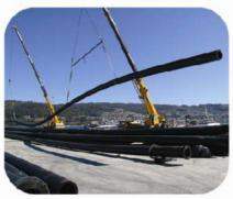
(3) The 65 m sections are transferred with a crane to the ramp area, from which they will be gently pulled down to the sea.
