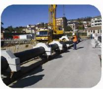
(5) Concrete weights are set every 2,5 m (covered with neoprene so that the pipes are not damaged) over the rails leading to the sea.
