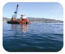
(8) The pipe sunk the previous day is refloated and placed on the platform with a crane. The 325 m section brought from Moaña beach is also placed on the same platform.
