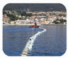
(9) Both sections are joined together with flanges placed at both ends, and floats are attached to them in order to make the sinking process easier.
