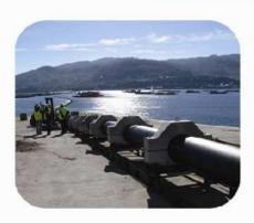
(6) The 65 m sections are gently launched to the sea. During this process they are welded to form new 325 m sections.
