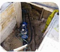
(11) The injection of potable water is controlled from land (opening valves). Once the pressures are balanced at both ends, potable water is injected into the pipe, pushing the pressurised air through the valve.
