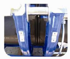
(2) Pipes are welded in **65 m sections** (approximate duration = 1,5 hours per welding).
